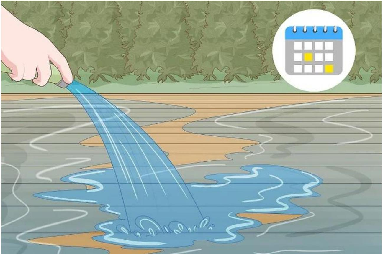
NB: Use a high pressure hose with a wide fan tip at pressures under 1500 psi. Remember to keep the hose at least 300 mm away from the surface when spraying.
